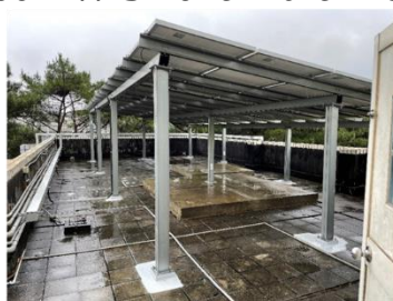
Installation of Solar Panel
